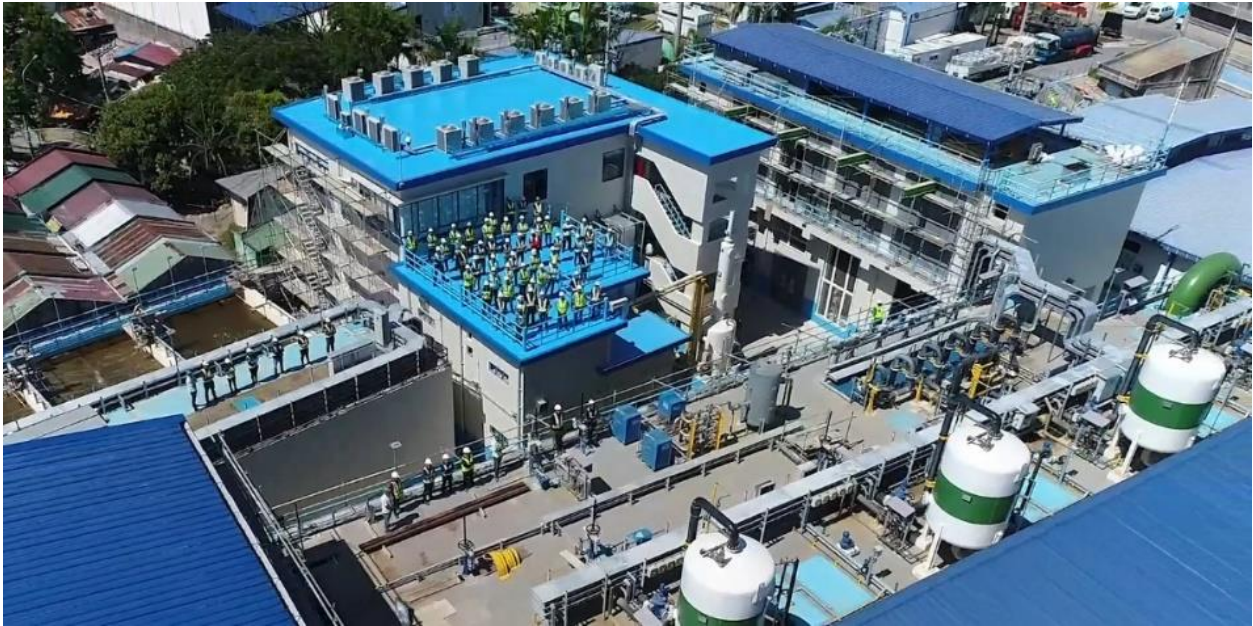
Figure 48: Al-Khobar Desalination Plant.
