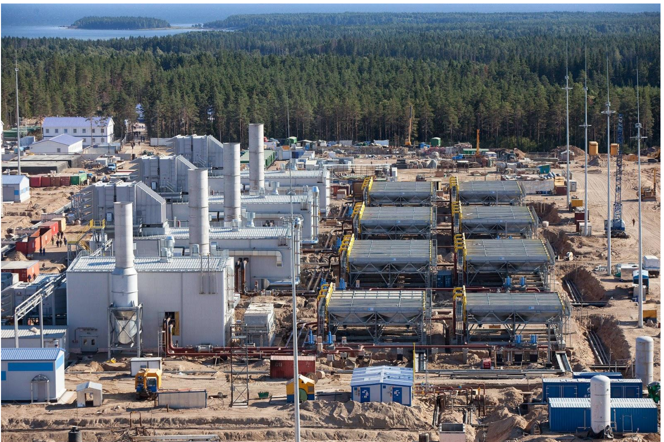
Figure 30: multiple unit compressor station [50]
